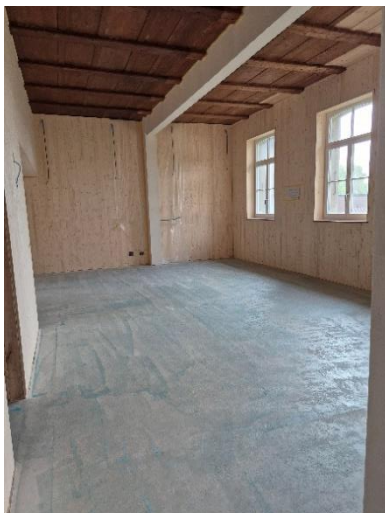
Essraum TS/Saal Restaurant
